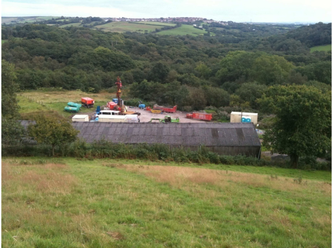
Figure 4: Drilling of Llangeinor 2 borehole
